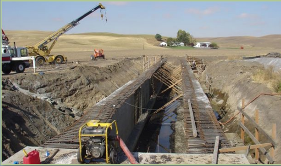
The box culvert at Genesee Junction will improve stormwater drainage.
